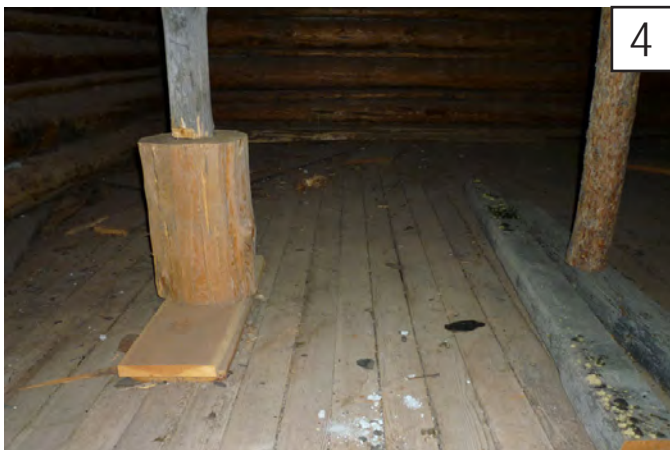
4 floor boards may show signs of wear and minimal deterioration.
