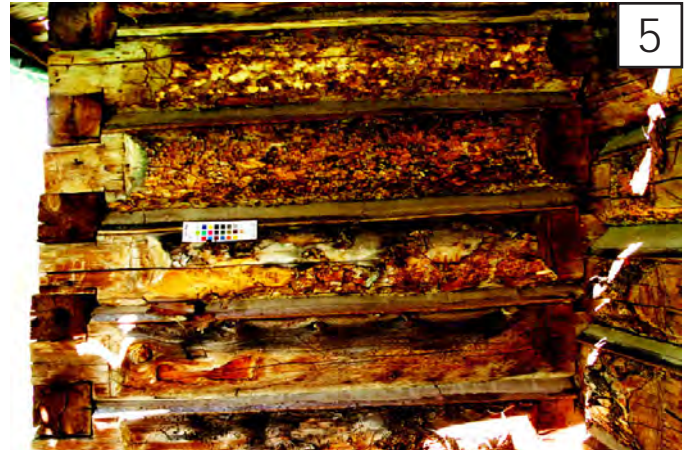
5 greater than 75% of total chinking material is present in the log joints.
