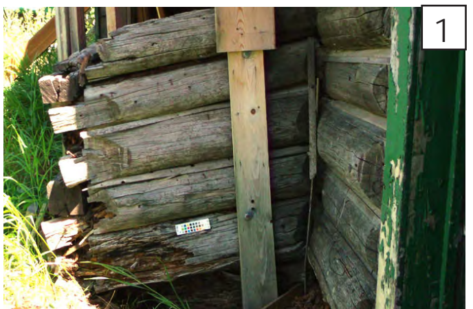
1 corners exhibit deterioration to the point of failure.
