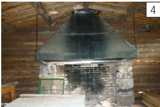
4 chimney condition exhibits some slight cracking or mortar loss but no major damage.
