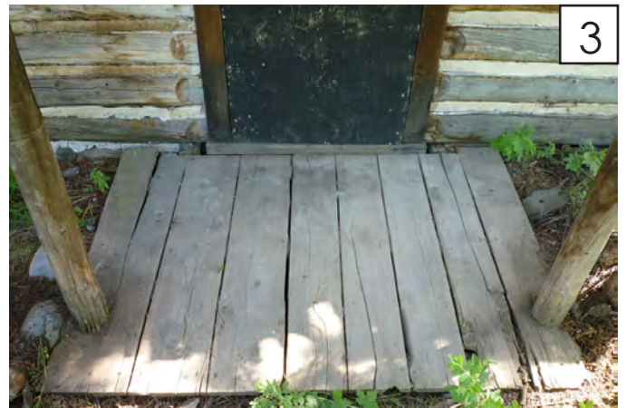
3 porch floor boards begin to exhibit slight warping and minor deterioration.
