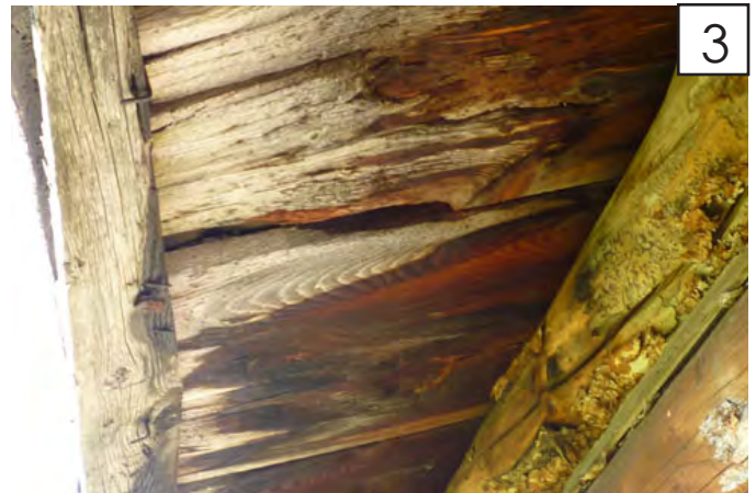
3 sheathing shows signs of water infiltration, minor rot and some splitting.
