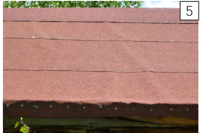
5 condition has no obvious condition or installation defect.
