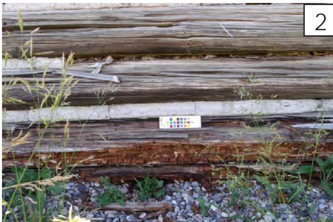
A 2 log is beginning to show rot and more severe deterioration.
