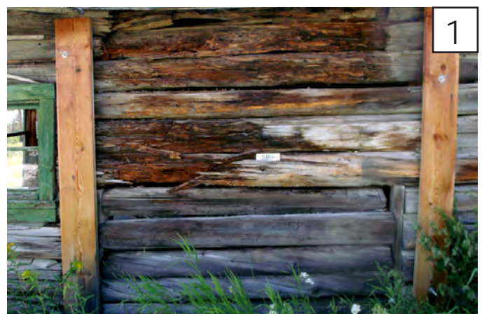
1 10% or less of total chinking material still is present in the log joints.
