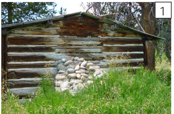
1 chimney condition denotes total failure and loss.
