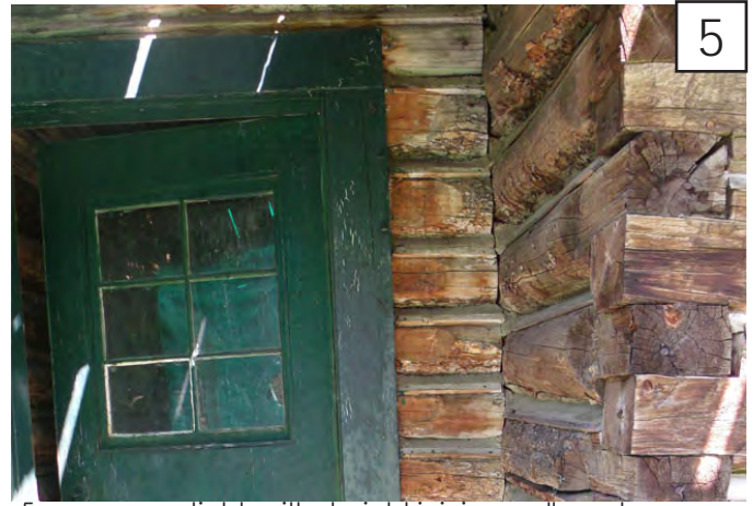
5 corners are tight, with straight joining walls and no open joints.
