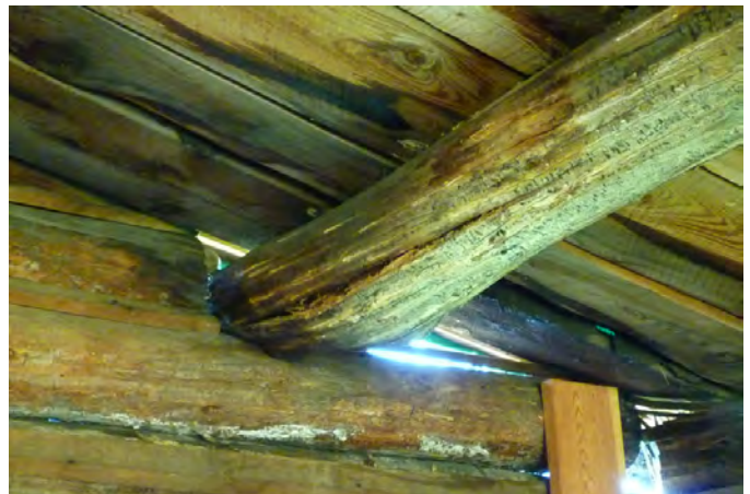
A purlin in poor, failing condition.
