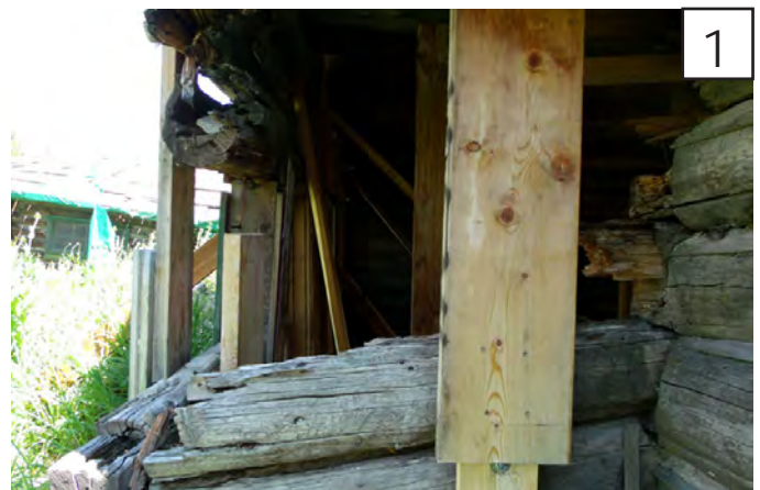
1 all logs rotted, deteriorated or missing, and are in danger of failure or are failing.
