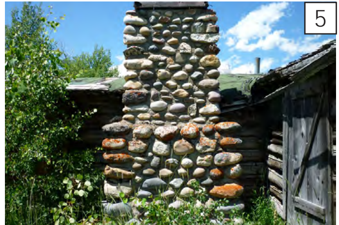
5 chimney condition exhibits no cracking or loss.
