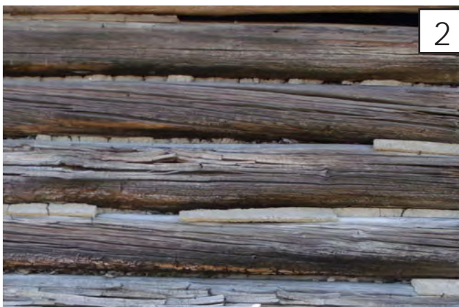
2 between 25 and 10% of total chinking material is present in the log joints.
