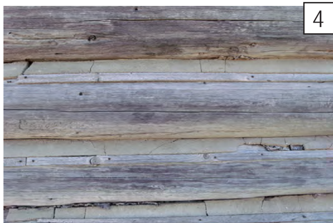
Mortar with lath stop.
