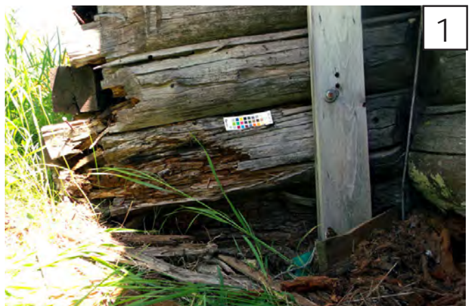
A 1 log is rotted, deteriorated or missing, and in danger of failure or are failing.
