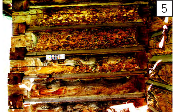
5 logs are tight and sound with minimal checking and no signs of rot.
