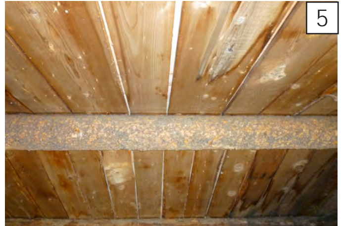
5 sheathing is sound and complete.
