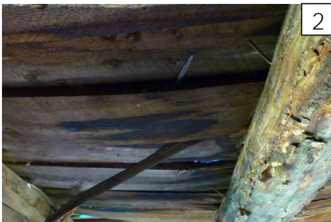
2 sheathing is more severely deteriorated, with evidence of rot and other decay.
