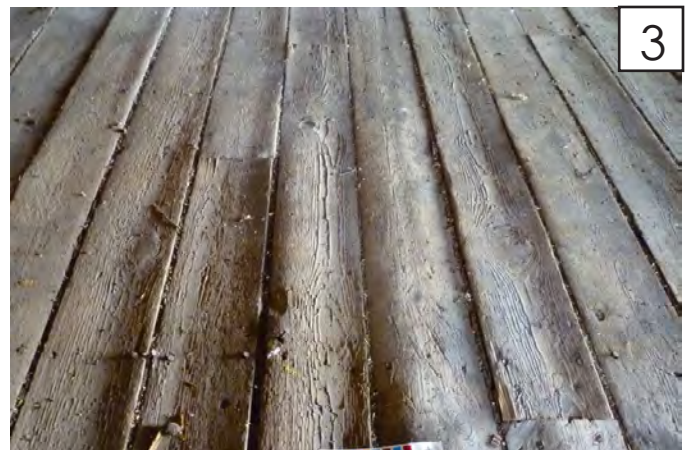
3 floor boards may be warped and moderately deteriorated.
