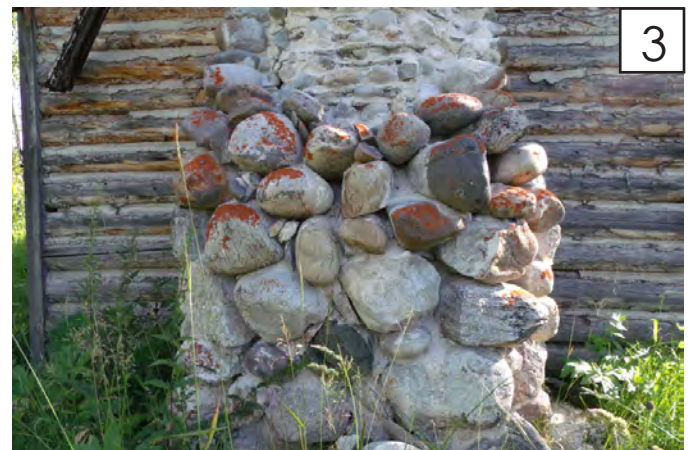
3 chimney condition exhibits major loss that does not affect structural integrity.
