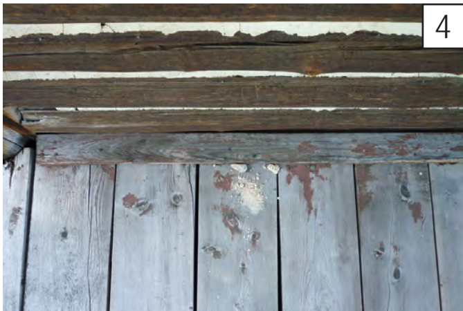
4 porch floor boards are basically straight and sound but may have some separation.
