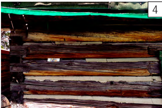
4 between 75 and 50% of total chinking material is present in the log joints.
