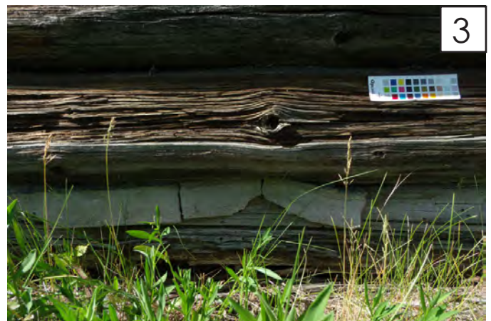
A 3 log has more advanced checking, splitting and signs of loss.
