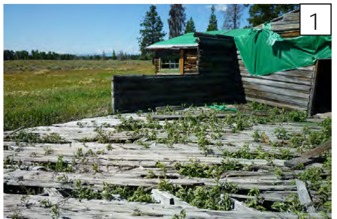
1 floor boards are extremely deteriorated, with material loss and failure.
