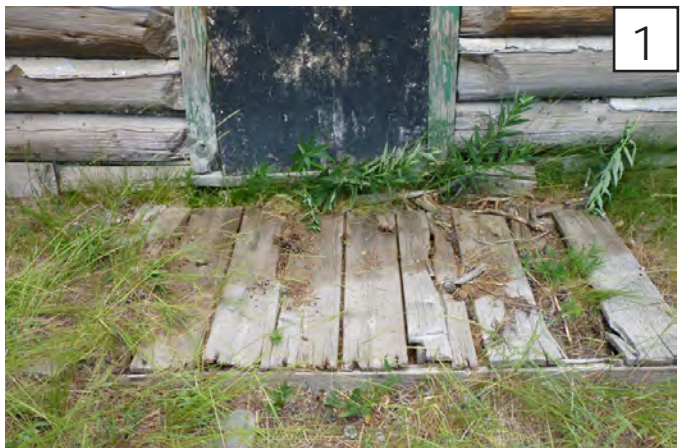
1 porch floor boards are warped, deteriorated, and have substantial material loss.
