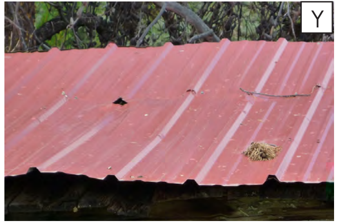
Roof deterioration evident.
