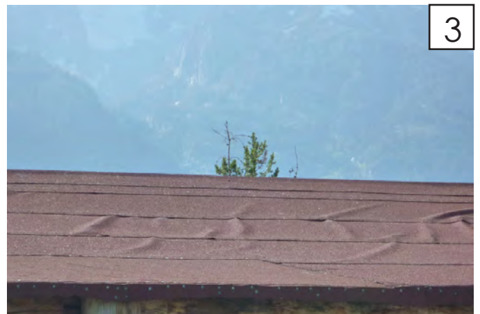
3 condition may be puckered, incorrectly installed, or beginning to show wear.
