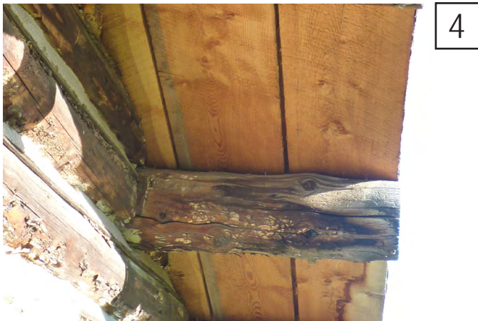
4 sheathing exhibits some minor signs of deterioration.
