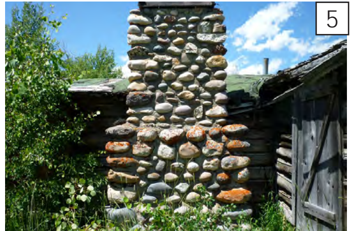
5 chimney condition exhibits no cracking or loss.
