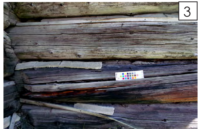
3 logs have more advanced checking, splitting and signs of loss.
