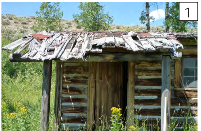
1 sheathing has reached the point of failure, material loss and extensive deterioration.
