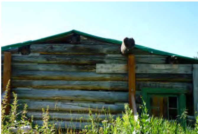
Three rotten purlin ends and one intact.
