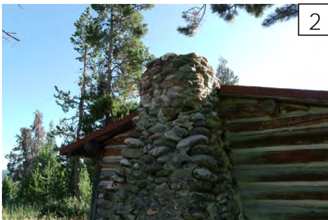
2 chimney condition exhibits major loss which penetrates to the interior of the structure.
