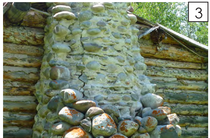
3 chimney condition exhibits loss that does not significantly affect structural integrity.
