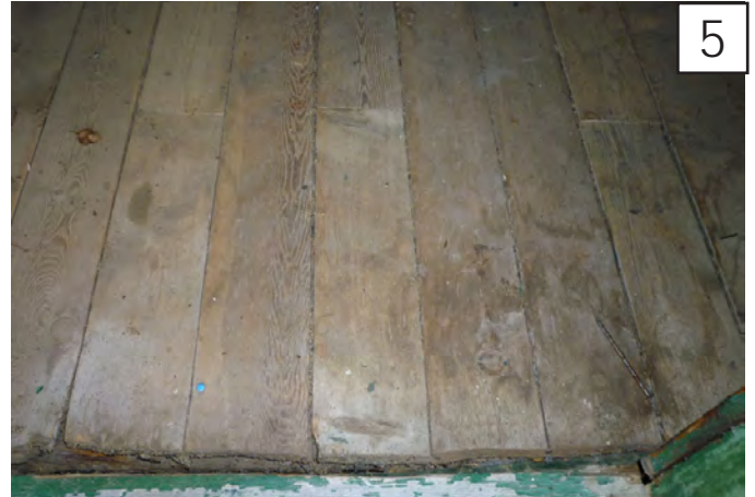
5 condition floor boards are straight and show no signs of damage or deterioration.
