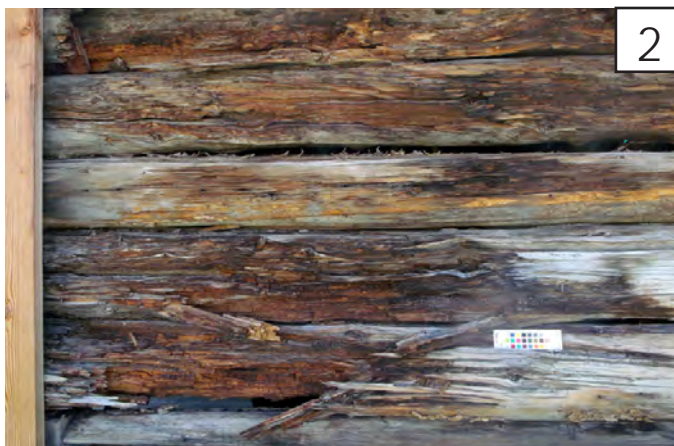
2 logs are beginning to show rot and more severe deterioration.
