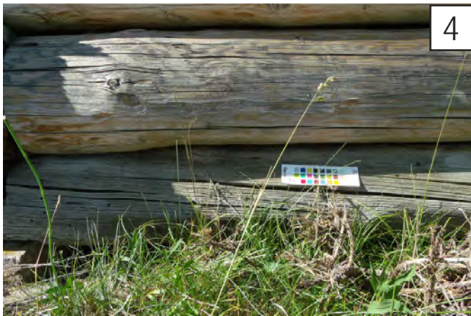
A 4 log may have more checking and some minimal signs of deterioration.
