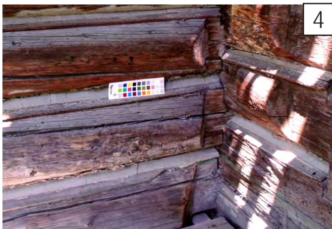
4 corners may have some slight openings, but remain straight and well aligned.
