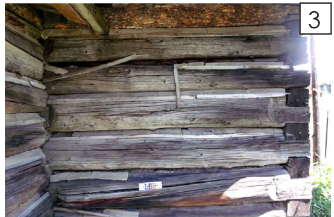
3 between 50 and 25% of total chinking material is present in the log joints.
