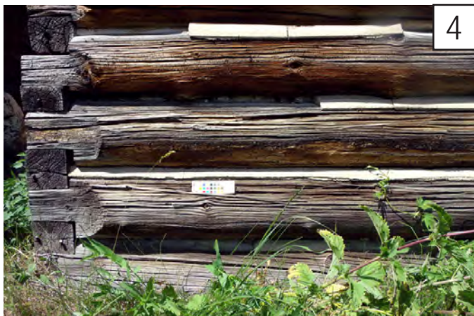
4 logs may have more checking and some minimal signs of deterioration.
