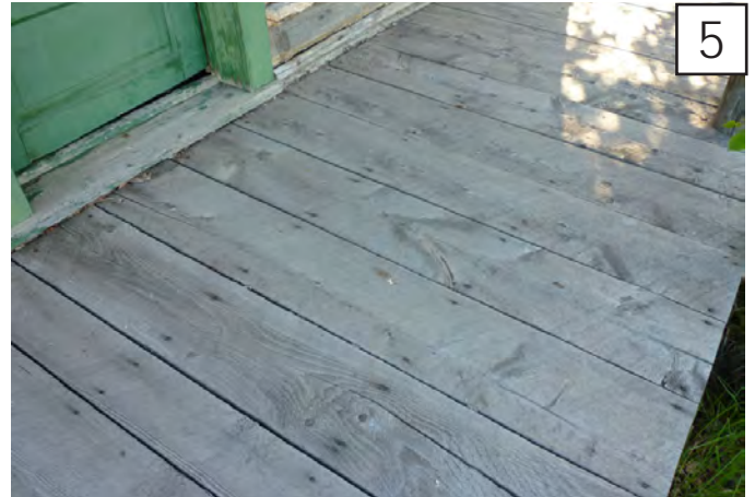
5 porch floor boards are straight and undamaged.
