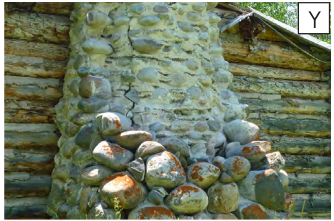
Cracking present.
