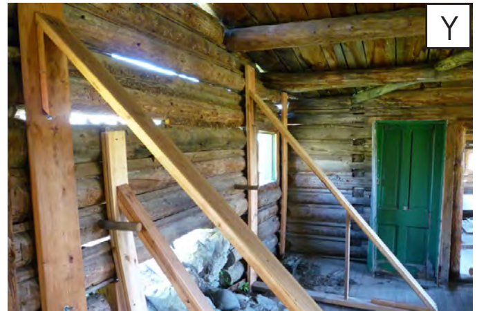
Interior stabilization present.
