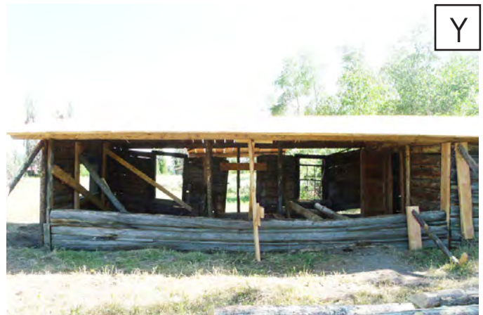
Deformation evident in the remaining lower portion of this wall.
