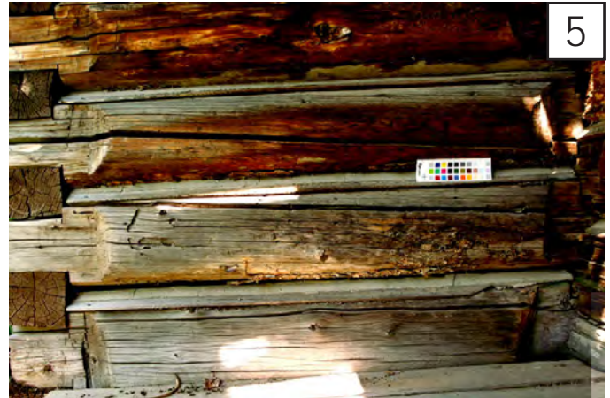
A 5 log is tight and sound with minimal checking and no signs of rot.
