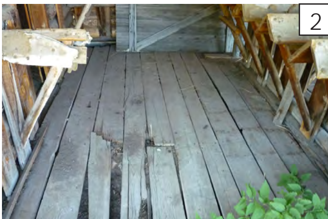
2 floor boards have areas of loss, broken boards, warping and are severely deteriorated.
