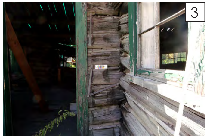
3 corners have separation in the log joints, the construction may exhibit slight displacement.
