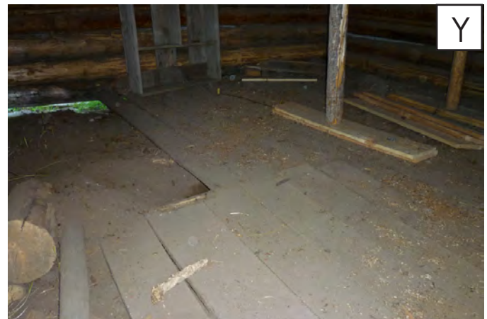
Floor deformation present.
