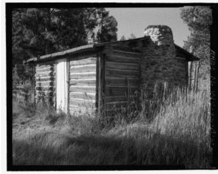
Figure 8- Bar BC Dude Ranch Cabin HABS Photograph
