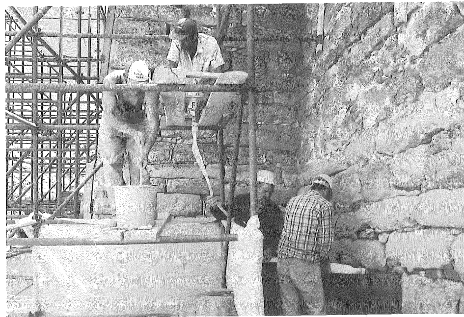
Fig. 16.3. Grouting the Early Phrygian Gate, 2003. Photo: Mark Goodman.
