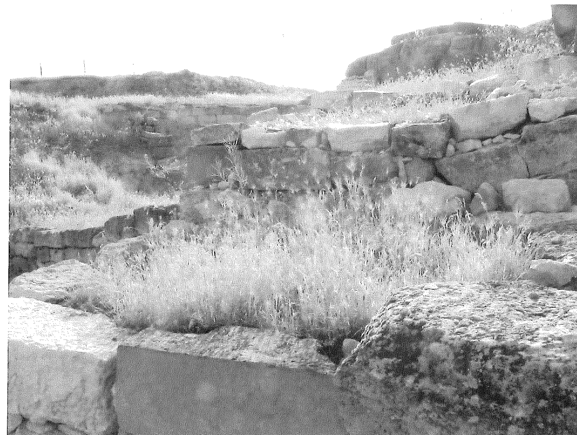
Fig. 16.10a–e. Installation of vegetative “soft” caps on north gate complex: (a) existing concrete cap prior to intervention; (b) capillary break layer; (c) filter layer; (d) completed “soft” caps; (e) view looking east of completed north gate “soft” wall caps. Source: Penn Architectural Conservation Laboratory.
