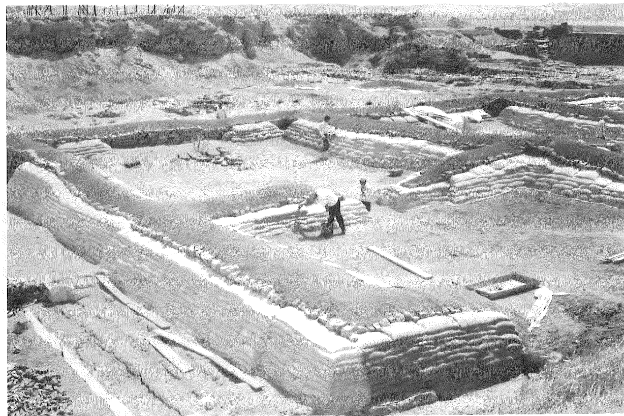
Fig. 16.4. General view of the Terrace Building with its temporary stabilization, 2001. Photo: Mark Goodman.
