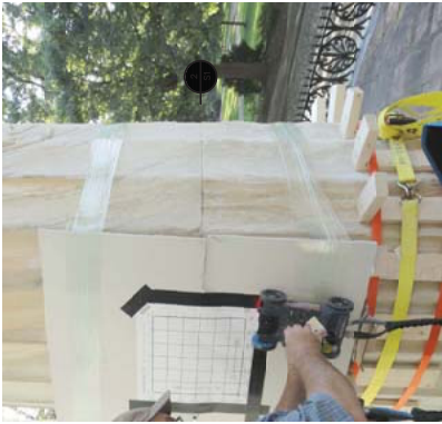
1 SURFACE PENETRATING RADAR TEST COLUMN 7 SOUTH ELEVATION
